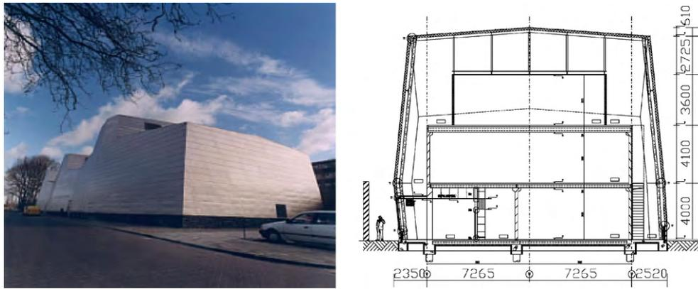
Fig. 1. (Top left) Impression of the Depot. (Top right) The box-in-a-box construction.
